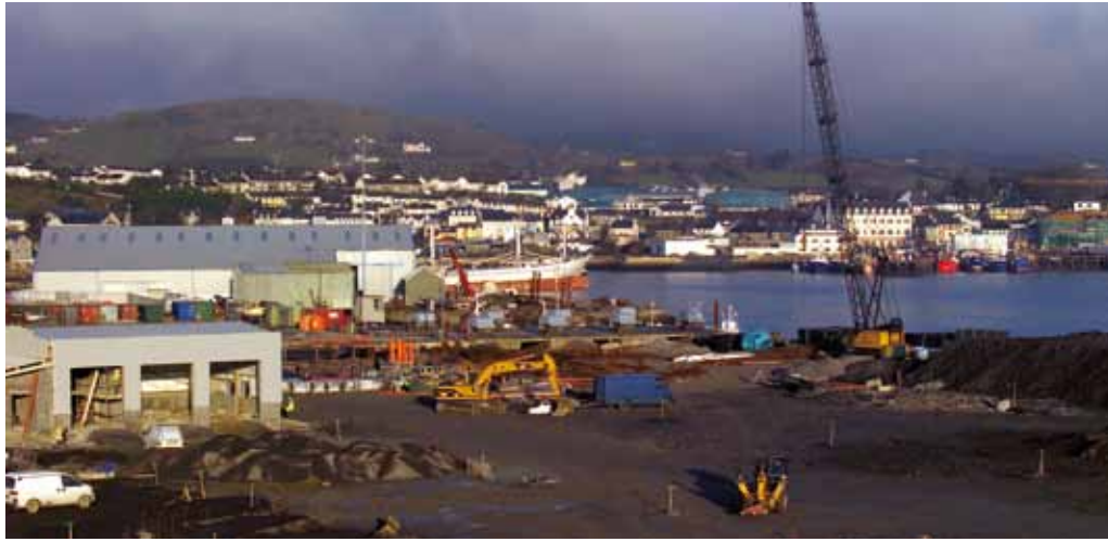
Killybegs Harbour Development, Co. Donegal, Ireland
