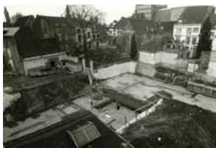
The construction of EIPA's extension.
